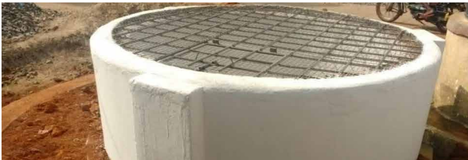
A refurbished well after removing the piles of plastic and cloth, and desilting and strengthening the walls
