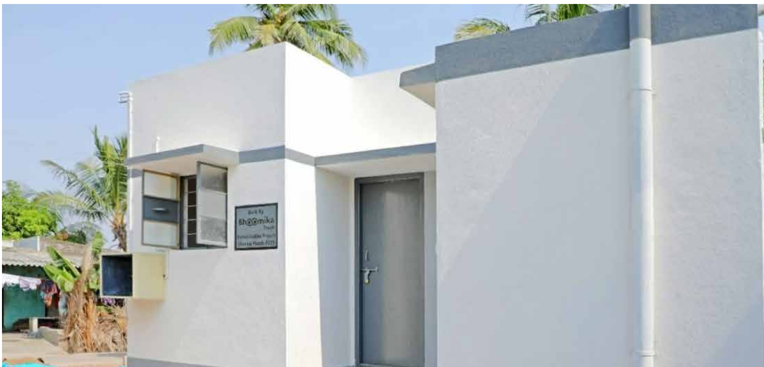
A resilient home built by Bhoomika, Manambathy Village
