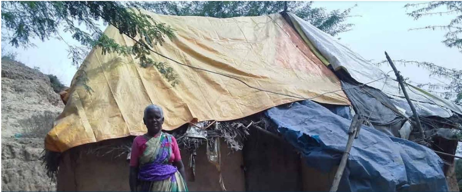
A house damaged by Chennai Floods, Manambathy Village
